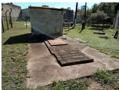
Foto 5 - Vista interna da EEE. Tecumseh Village
